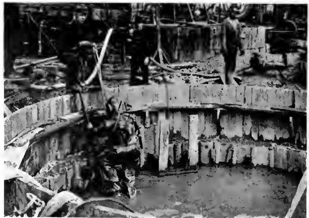
DIVER ENTERING CYLINDER TO EXAMINE ROCK SURFACE
